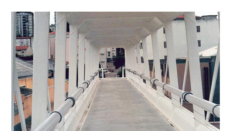
Gurit engineered a composite footbridge span for installation in Lisbon for the 1998 EXPO. Two of the bridges span across roads, and the third crossed a railway line. Design was carried out to Portuguese codes, including seismic load cases.
