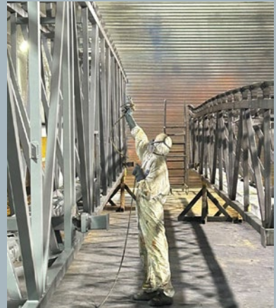
Airless painting is now used to protect the steel structure and frames, reducing pollutants, material use and waste (China)
