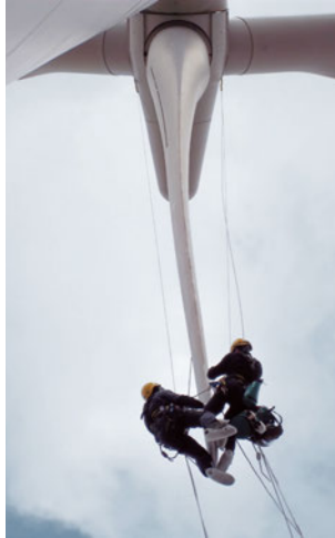
Repair works on a wind blade
