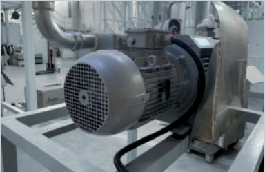
Replacing the old pumps by new ones which won’t require water to work and therefore won’t produce polluted water
