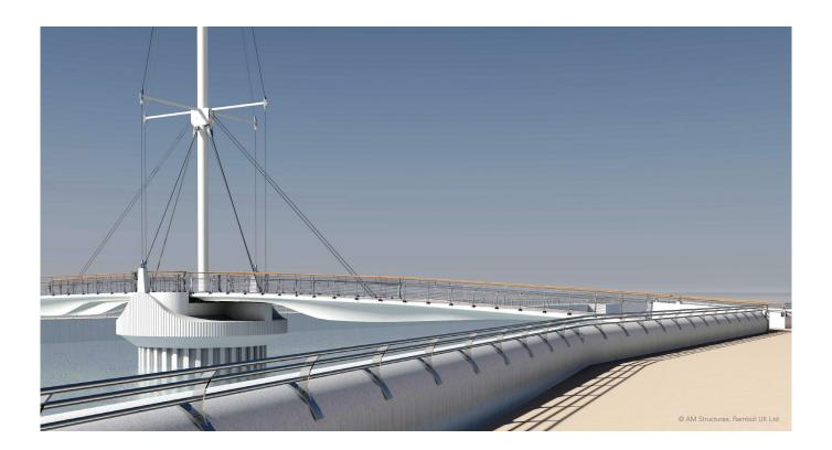
Ramboll approached AM Structures in early 2009 to review the concept of the bridge deck construction and to provide feedback on the construction and weight estimate for the FRP decks. AM Structures asked Gurit to review the structure of the bridge, and initial studies confirmed that the bridge concept was feasible with some minor changes in the geometry, and that the FRP decks would result in considerable savings compared with a steel structure.
