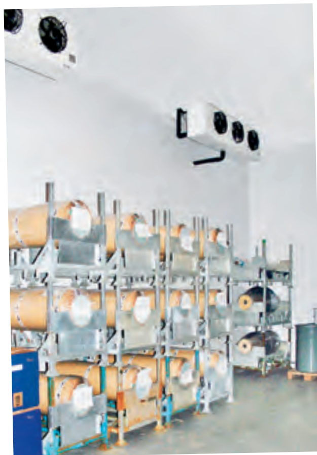
Shut the coolers off! The next generation of Gurit prepreg does no longer requires chilled storage.
