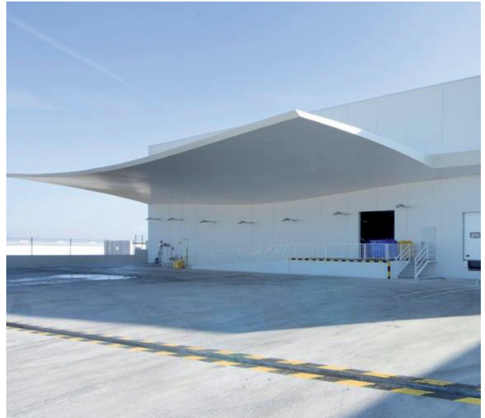
Above: The 340sqm, curved, self-supporting canopy over the loading dock
