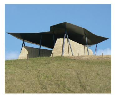
Definition of the material cost as a custom design variable within the software allowed for driving the optimisation towards minimising cost rather than the more usual objective of minimising weight. Finally an optimum was found between minimum material cost, and structural integrity, while realising the artistic intent.
