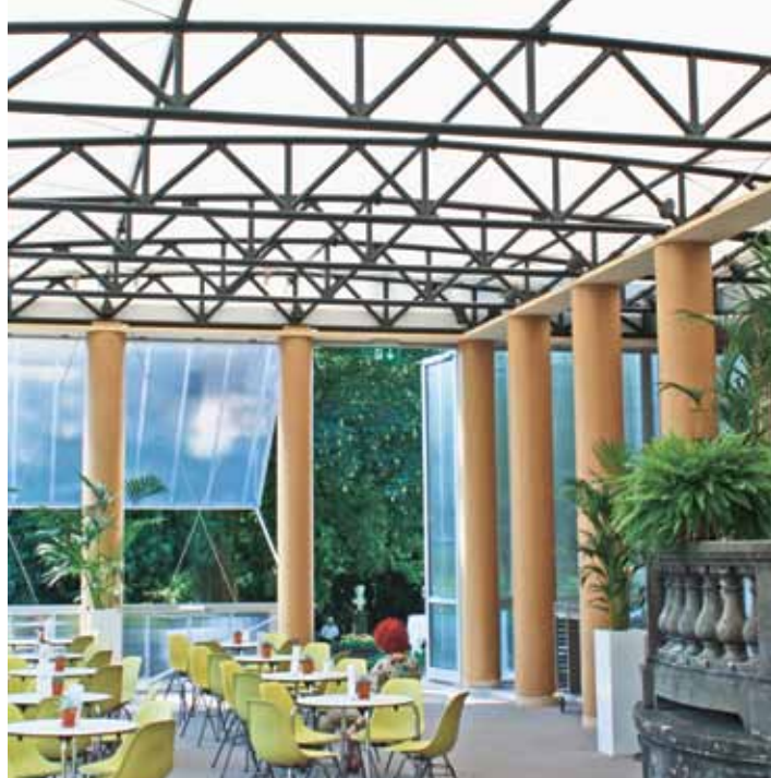
The carbon cross beams that support the tent roofing of the Summer Pavilion rest on cardboard columns which were only «unveiled» when the roof was up. Festival goers and park visitors alike hope that the lightweight pavilion will be put up again next year.
