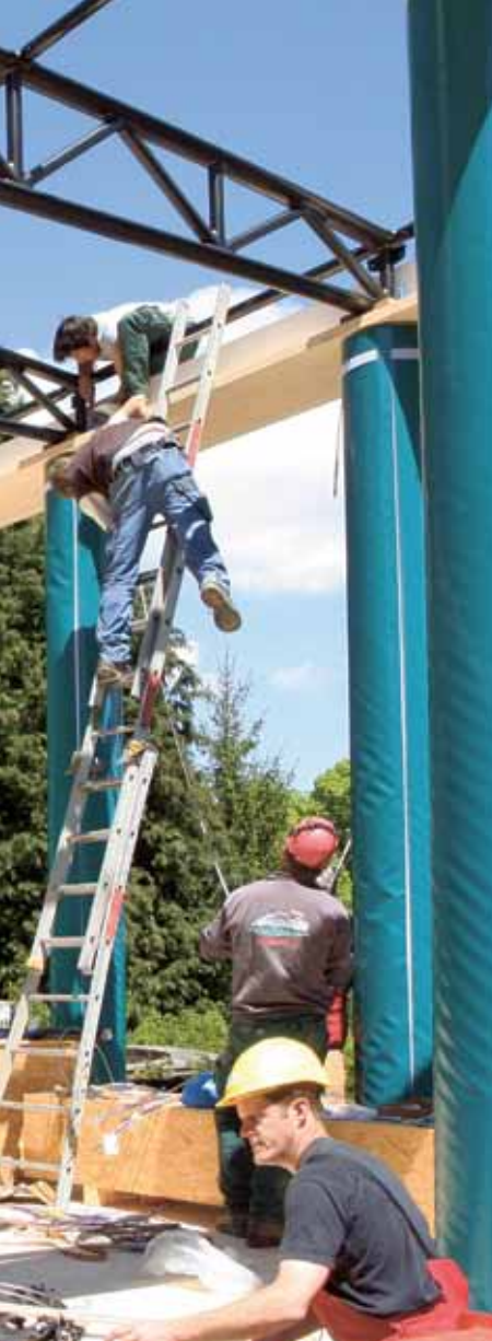
The carbon cross beams that support the tent roofing of the Summer Pavilion rest on cardboard columns which were only «unveiled» when the roof was up. Festival goers and park visitors alike hope that the lightweight pavilion will be put up again next year.
