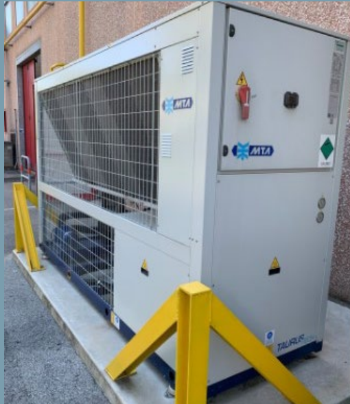
Upgrading heat exchange units to reduce energy consumption
