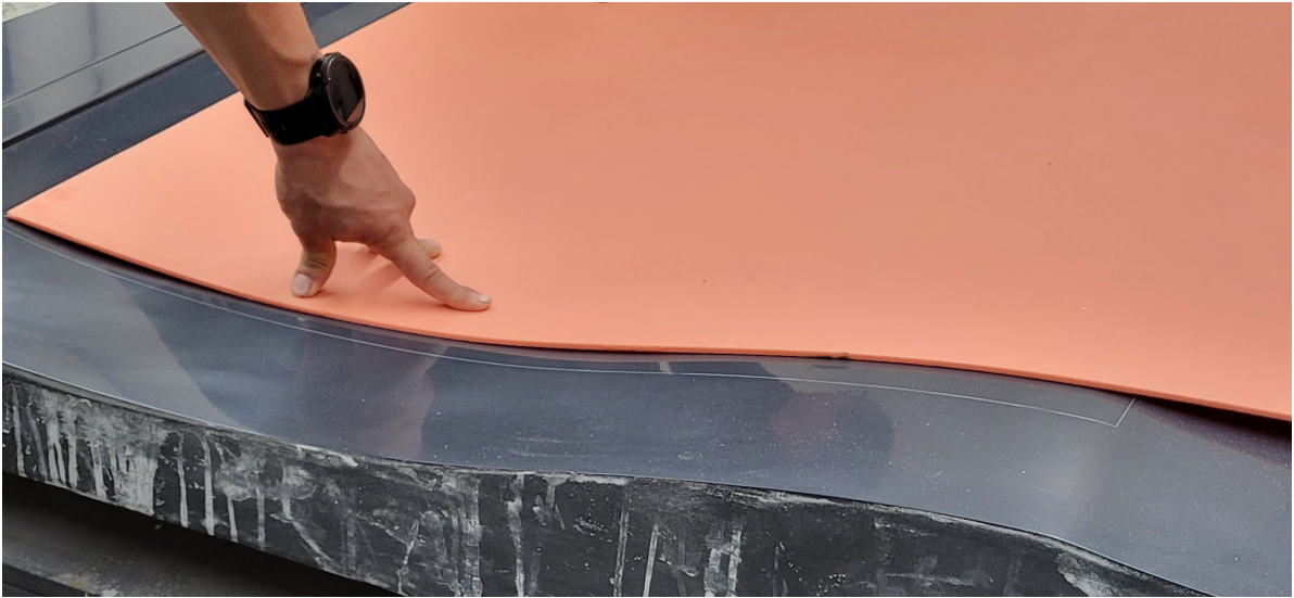
Dry test of the positioning of I-60 Corecell™ in the mould
