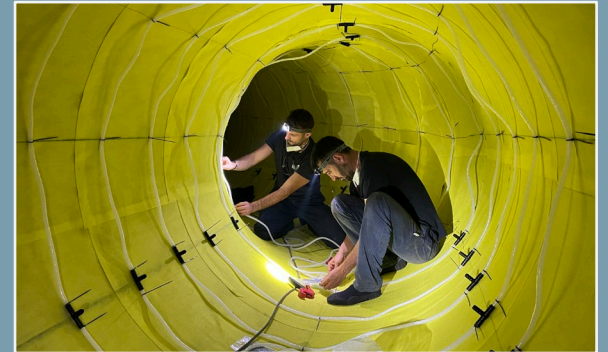
Water pipes retrofit/repair with composite materials
